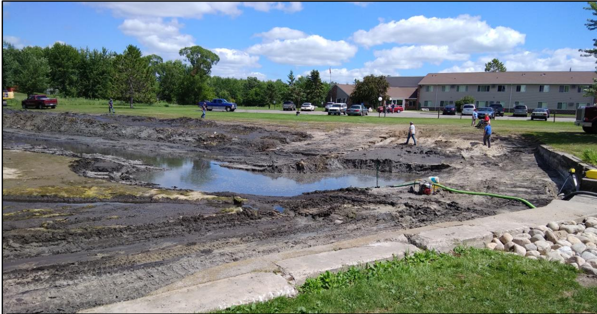
Excavation within the pond along Clear Brook in the town of Clearbrook (the work that was permitted by the DNR)
